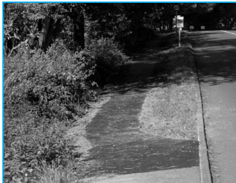
The rebuilt footpath alongside 2nd fairway North Downs G. C.
